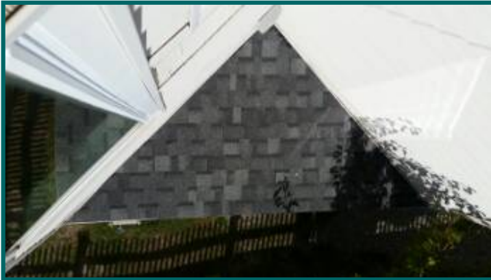
shingled roof at lower side area
