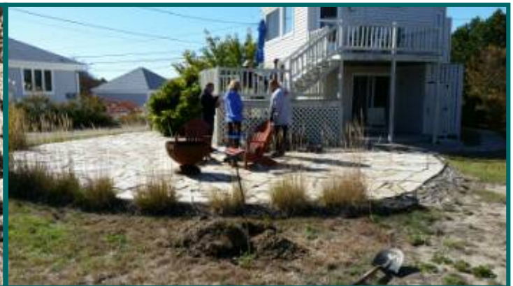
Leach field in foreground, septic tank in background
