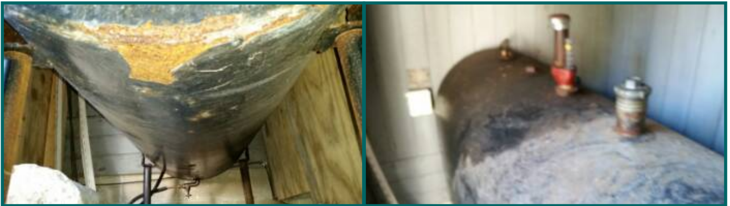
Underside of oil tank
