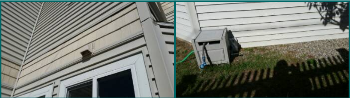
First floor bath fan termination.
