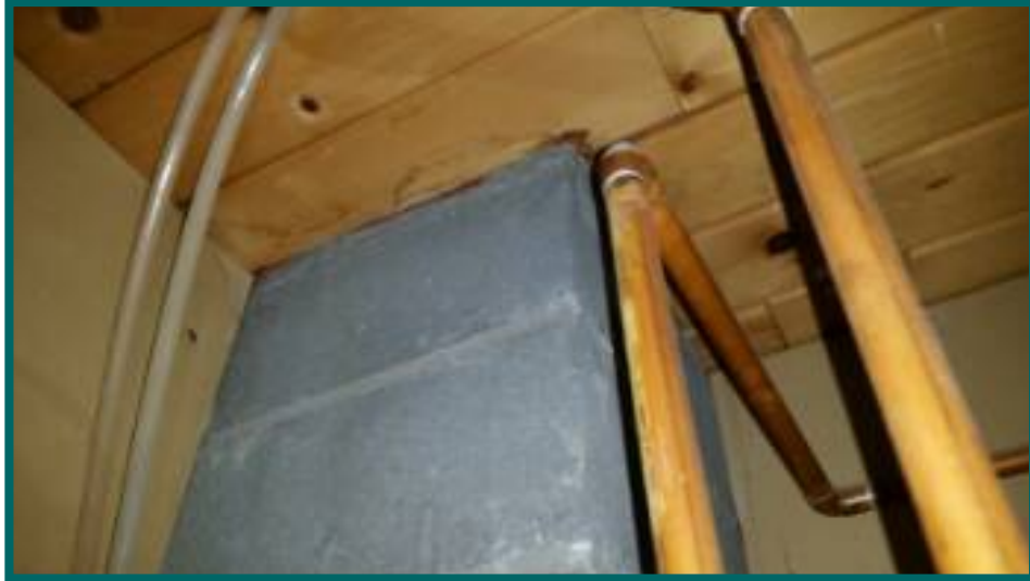
Basement ceiling around chimney
