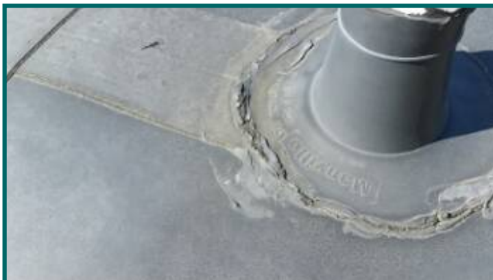
crack sealant on second roof vent stack
